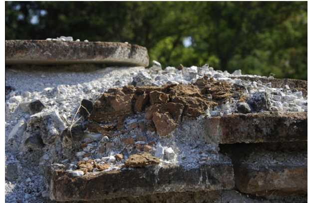
Fig. 3. State of preservation of building materials (mortars, bricks).
