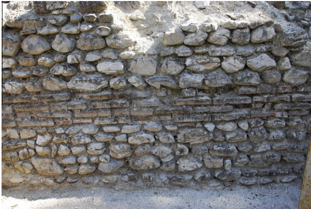
Fig. 1. Masonry type of Odeion (opus-mixtum).
