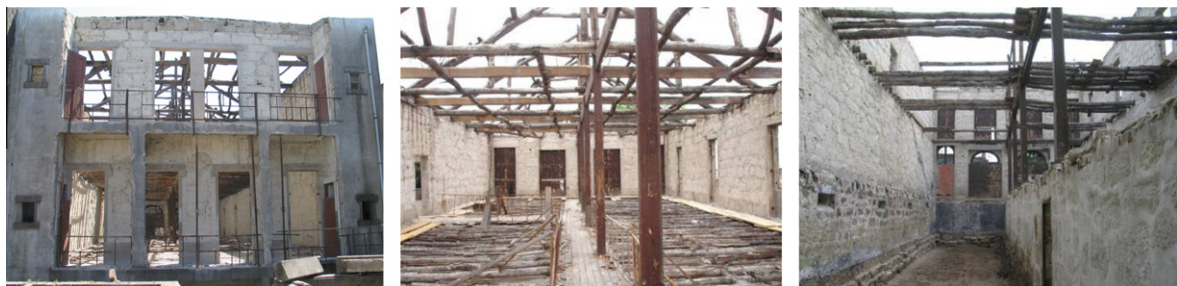
Fig. 1. Rehabilitation works in the studied building.
