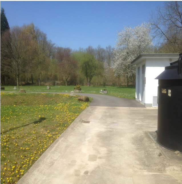
Fig. 1. Exterior view of unmanned pumping station. As can be seen, it sits in a field.
