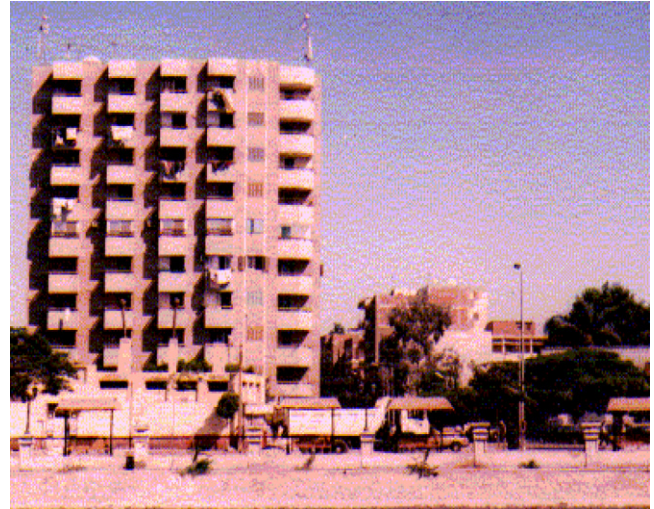
Fig. 1. The mobile phone base station antennas upon the building for agricultural professions.
