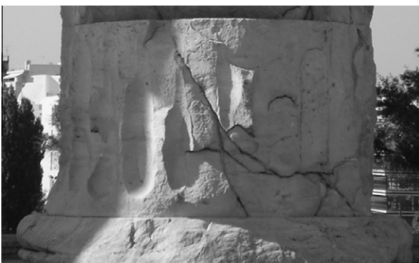
Fig. 2. Photo of the bottom cracked drum of a column at Olympieion temple in Athens.
