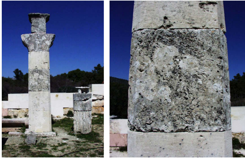
Fig. 1. An overview of a restored pillar from Avaton of the Epidauros Archaeological site, exhibiting the coexistence of ancient (Kenchrean porous stone) and new material [1].
