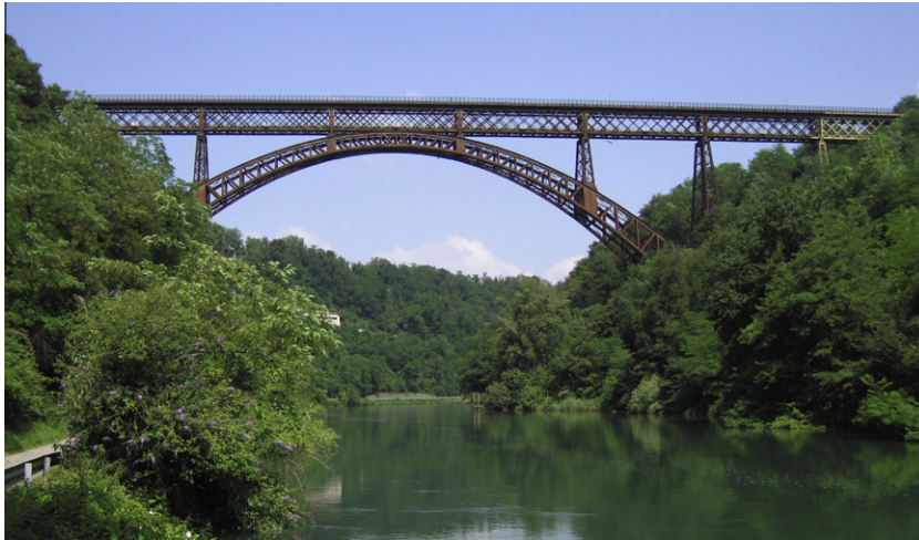
Fig. 1. View of the Paderno iron arch bridge (1889).
