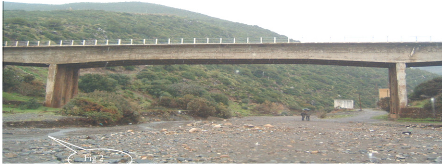
Fig. 1. Overview of the bridge.
