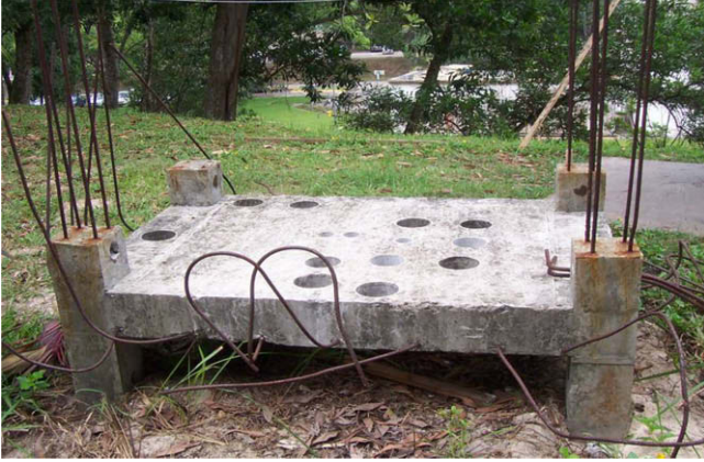
Fig. 1. RC model structure exposed to natural environment.
