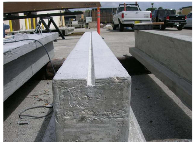
Fig. 3. Typical NSM groove.
