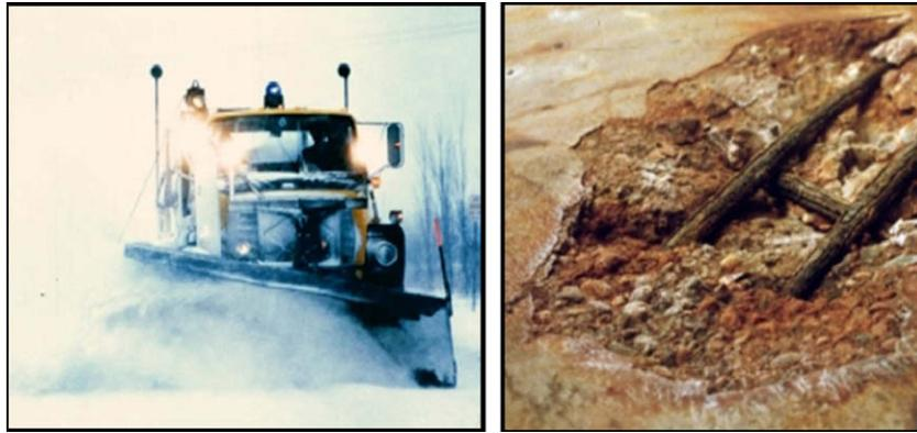
Fig. 1. Winter conditions and corrosion of steel reinforcement typical to many bridges in Canada.
