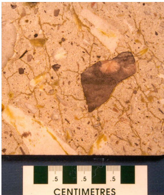
Fig. 1. Thin and isotropic cracks in ASR-affected dam concrete as highlighted with epoxy impregnation.
