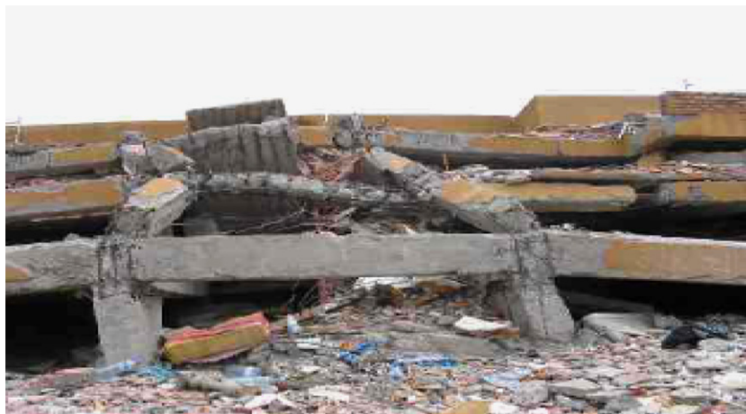
Fig. 1. Failure of a structure under the effect of the seismic action [1].
