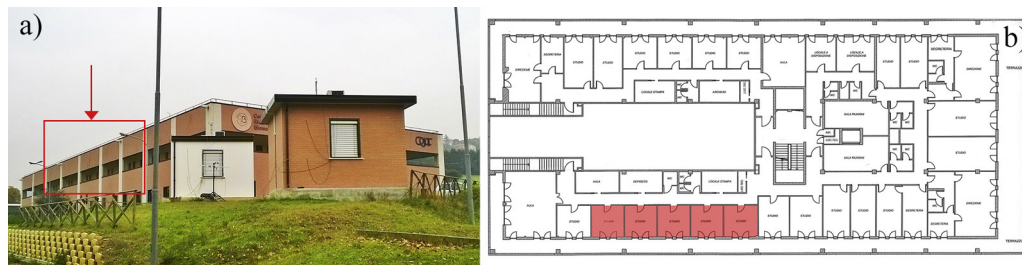
Fig. 1. (a) Picture and (b) plan view of the monitored institutional building in Perugia, Italy.
