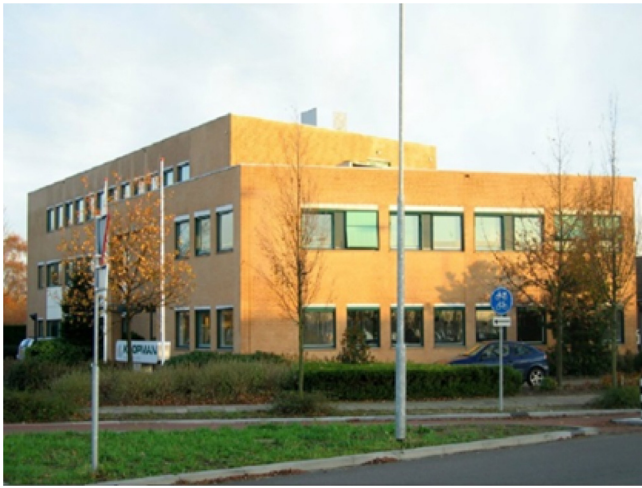
Fig. 1. Test-bed office building.
