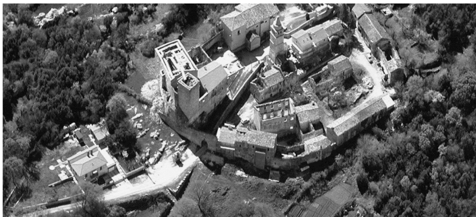
Fig. 1. Aerial view of the Krsan Castle [18].
