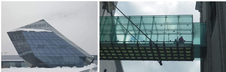
Fig. 1. Office building in Austria and shopping mall in Germany (photo by A. Lechowska).
