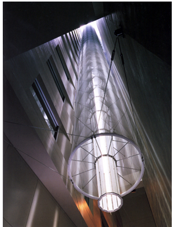
Fig. 1. A 14-storey height sun pipe.
