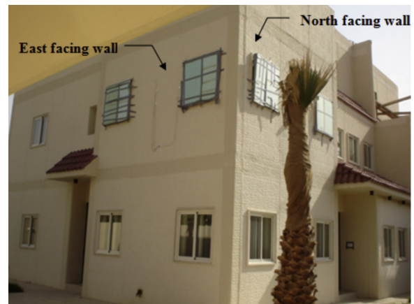
Fig. 1. Outside view of the instrumented walls of the building.
