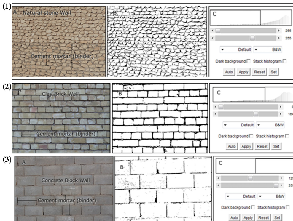
Fig. 1. External wall fabric using natural stone, clay brick, and solid concrete block.
