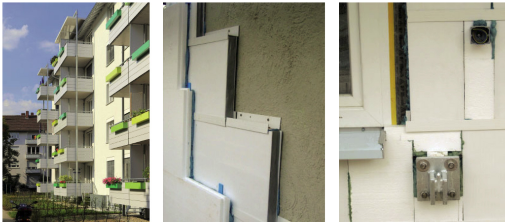
Fig. 1. VIP used in the retrofitting of a multi-family building in Karlsruhe, Germany. The 40 mm thick VIP was attached to the façade in a rail system and covered on the exterior by 50 mm EPS. The aim of the design was to maximize the surface covered by VIP.
