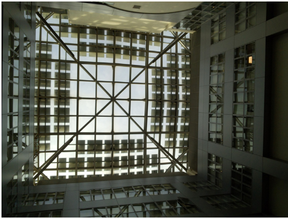
Fig. 1. Photo of the skylight.
