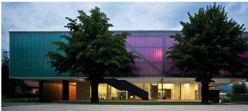
Fig. 1. Example of a building with PC façades (DAP Studio in Bergamo, Italy. Courtesy of SEP).
