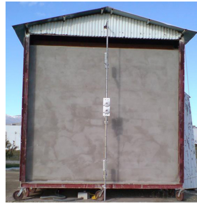
Fig. 1. Exterior view of the wall tested.
