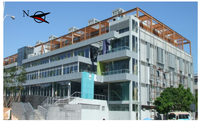
Fig. 1. The tested office building in Shenzhen.
