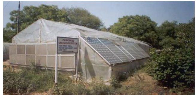
Fig. 1. Picture of experimental set-up at solar energy park, IIT Delhi campus.
