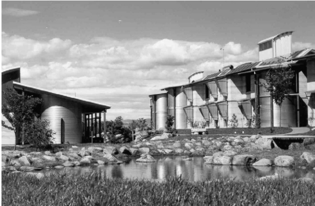
Fig. 1. Northern aspect of rammed earth office building (right of figure).
