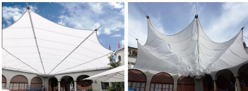
Fig. 1. Most adaptable fabric structures are only prestressed, and thus functional, in one configuration (left) and transform by folding the fabric. However, during this process the prestress is usually lost resulting in the fabric becoming slack (right) [© Kugel Architekten ( http://www.kugel-architekten.com )].
