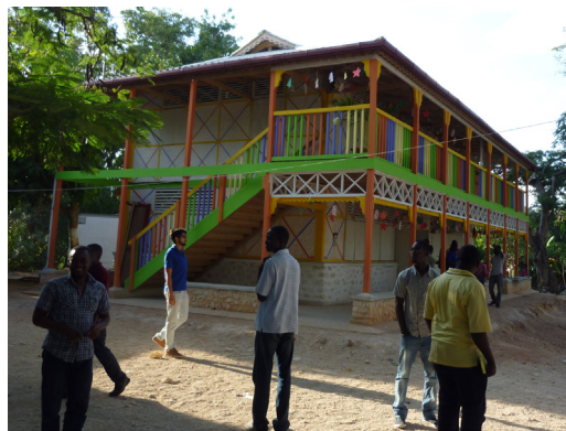
(c) School two-storey project in Grand Boulage, (Entrepreneurs du Monde)
