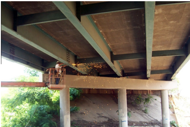
Fig. 1. I-40 westbound bridge over 4th Avenue in Knoxville, TN.
