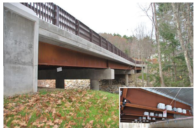
Fig. 1. Powder Mill Bridge.
