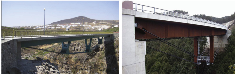
Fig. 1. Two recent examples of under-deck cable-stayed bridges with composite decks: (a) San Miguelito creek footbridge in Queretaro (Mexico) designed by Carlos Fernandez Casado SL and completed in 2008 (photo courtesy of Arturo Perez Aguilar and Christian Balcazar Benitez, Mexpresa) [7]; (b) Okuno bridge in Japan (photo courtesy of Toshiyuki Nakagawa) [8].
