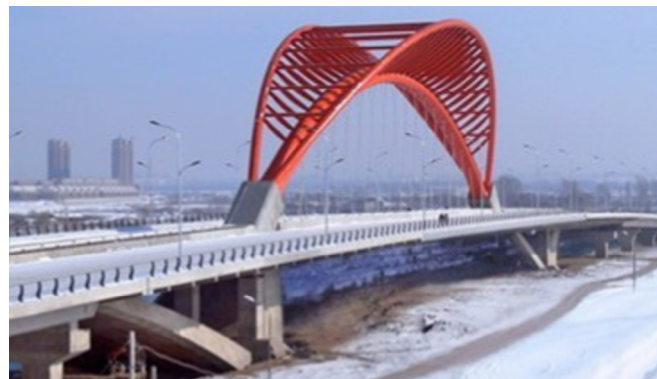
(c) Overview of the bridge
