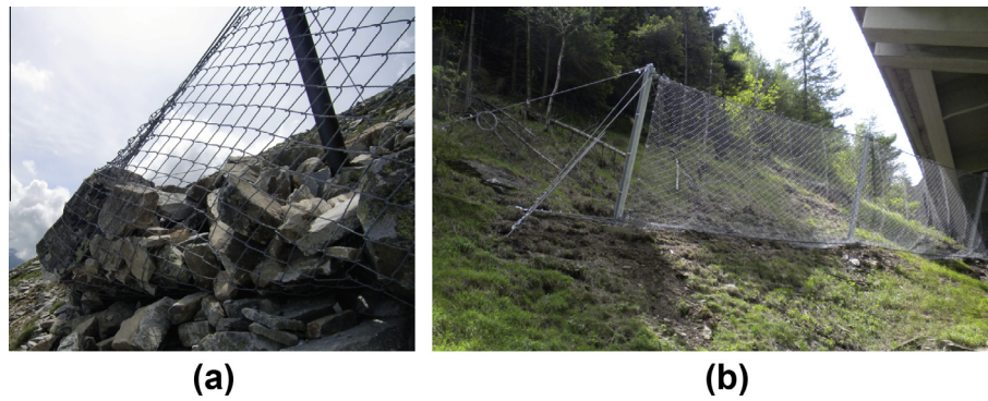
Fig. 1. Rockfall protection barriers: (a) wire-rope chain link net as part of a rockfall barrier impacted by a rock avalanche and (b) double chain-link interception structure as part of a rockfall barrier.
