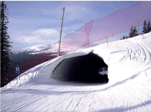
Fig. 2. Corrugated flexible culvert for a ski slope in Åre, Sweden.
