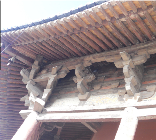
Fig. 1. The layered beam structure in Yingxian pagoda.
