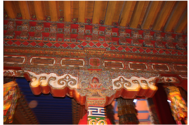
Fig. 2. The layered beam structure in Tibetan ancient architecture.
