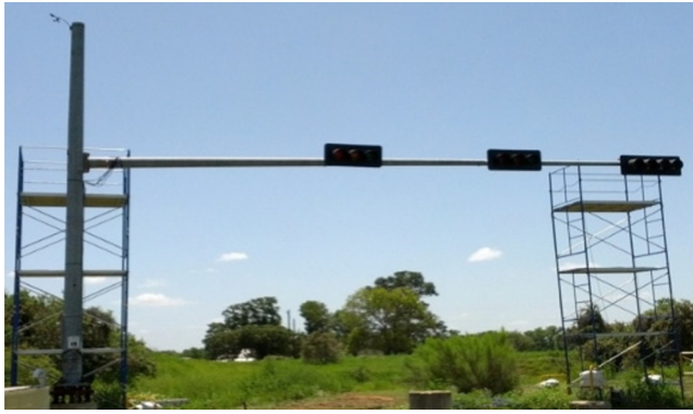
(a) Full-scale traffic signal support structure
