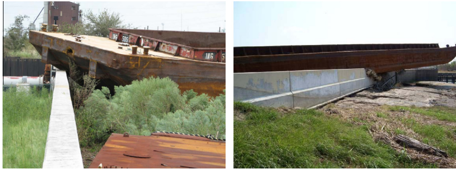
Fig. 1. Aberrant barges that impacted New Orleans area floodwalls during Hurricane Katrina. Source: U.S. Army Corps of Engineers.
