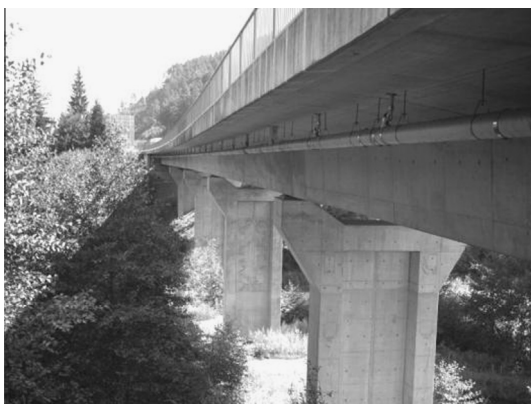
Fig. 1. Example of a viaduct supported by I-shaped columns.
