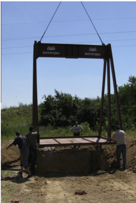
Fig. 1. Test frame and the foundation pit.
