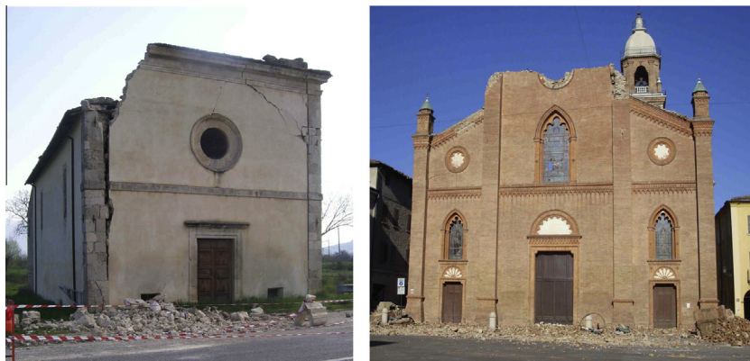
Fig. 1. Seismic failure mechanisms in masonry churches: Overturning of the façade (left), overturning of the gable (right).
