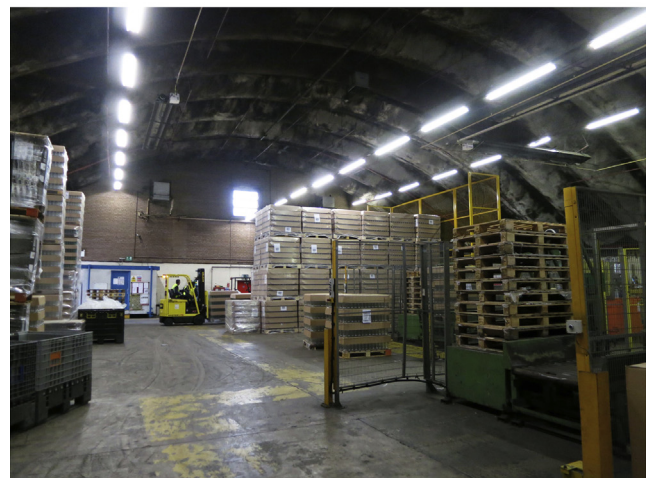
Fig. 2. Formwork [5] (top) and current state in 2013 (bottom) of the shell of the Chivas Distillery Warehouse, now Chivas Central Bottling Hall and despatch warehouse, Scotland, ca. 1959, by James Waller et al., with 30.5 m spans and thickness of 6.4 cm. Photo (bottom) courtesy of Chivas Brother Ltd.
