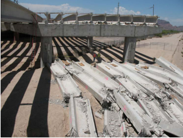
Fig. 1. Stability failure of precast prestressed AASHTO Type-V girders during the construction of the Red Mountain Freeway in Arizona [1].
