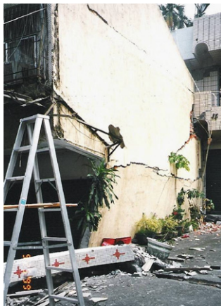
Fig. 2. A confined masonry building damaged along the out-of-plane direction of walls during Chi-Chi Earthquake, 1999.
