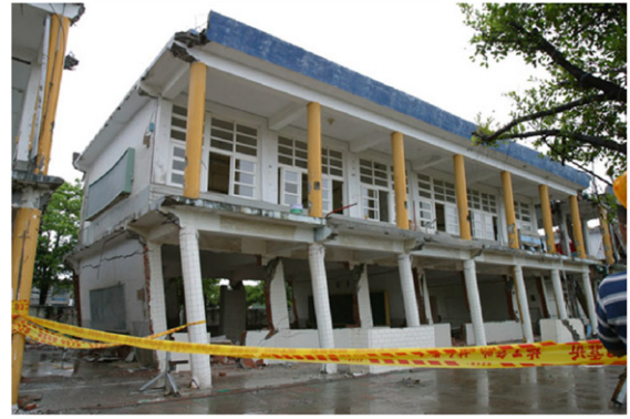
Fig. 4. Final stage of a specimen from in-situ tests on school buildings.
