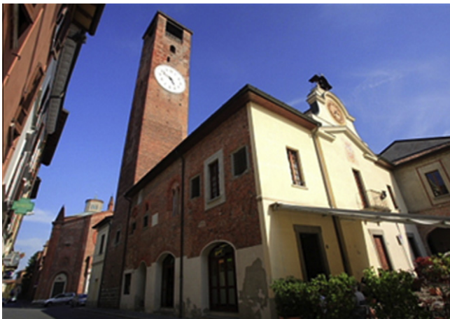
Fig. 1. North–west view of the medieval civic tower of Soncino (Cremona, Italy).
