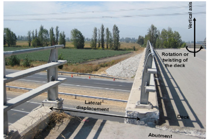
Fig. 1. Typical damage of overcrossings after the Chile earthquake of February 27, 2010.
