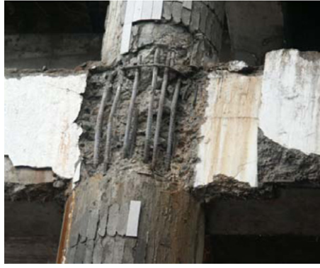
(a) Joint shear failure.
