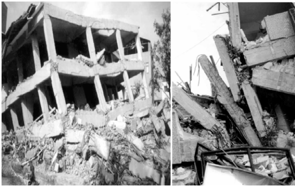
Fig. 2. Typical beam–column joint failures (Turkey earthquake).
