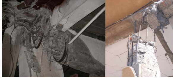
(b) Inadequate reinforcement anchorage.
