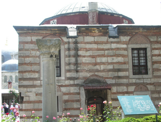
Fig. 2. Old combined masonry construction in Istanbul, Turkey.
