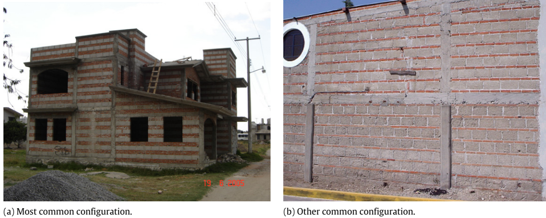
Fig. 1. Combined and confined masonry construction currently built in Mexico.
