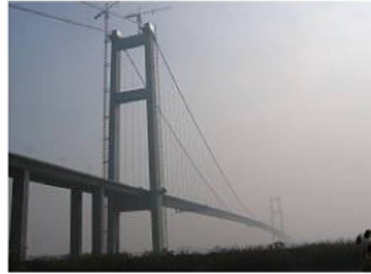
Fig. 1. Runyang suspension bridge (RSB).
