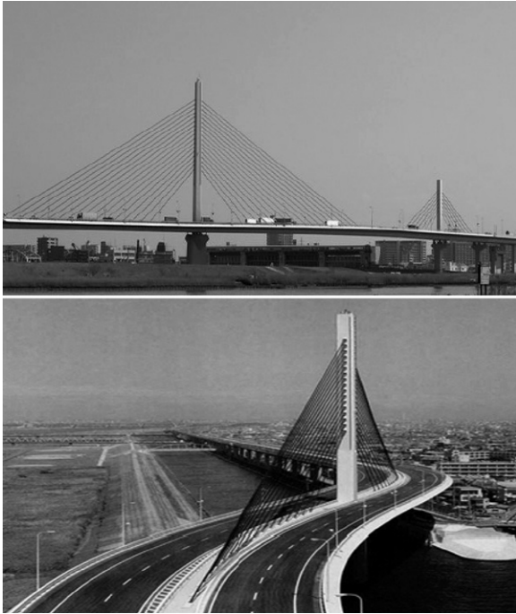
Fig. 1. View of the Katsushika–Harp bridge.
